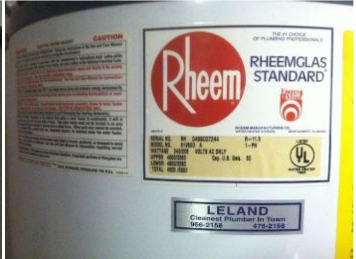
81 gallon HW heater in garage -replace with 40 gallon unit at re-piping time.
