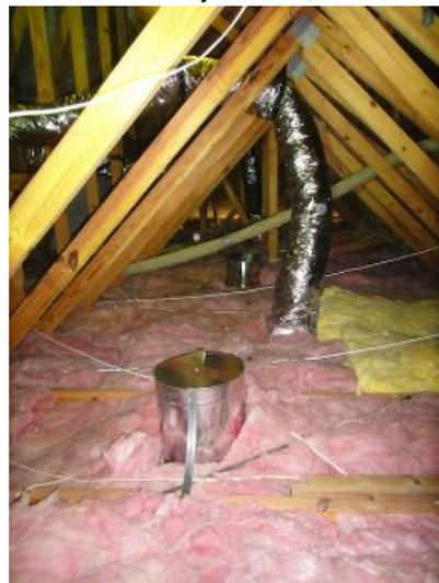
Showing new can light covers and new ductwork - before new insulation added.
