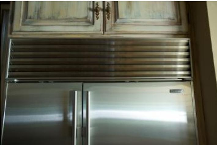
I could not remove this fridge cover, it is full of dust, needs removal and the coils vacuumed out.
