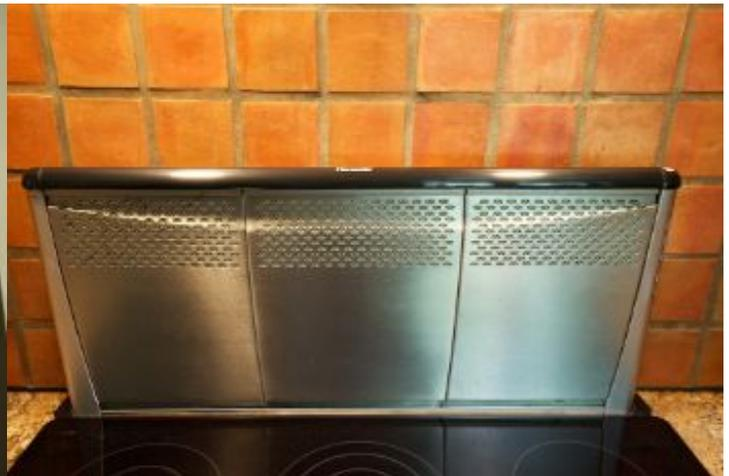
Stove vent clogged with grease, clean and check for venting.
