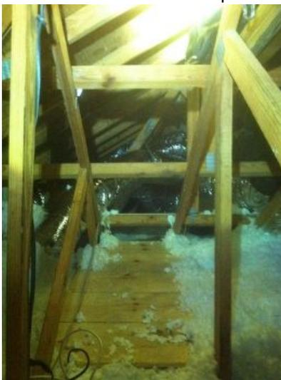
New insulation and walkway over wires resolved multiple issues.
