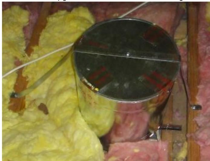
Showing new can light covers and new ductwork - before new insulation added.
