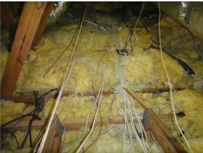
Unprotected wires and scant insulation - upgraded.
