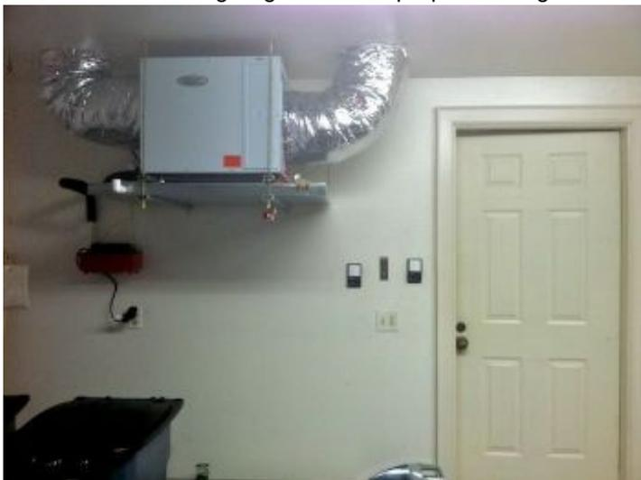
Household dehumidifier installed in garage will address moisture issues even if the A/C is not running as in the cooler months.
