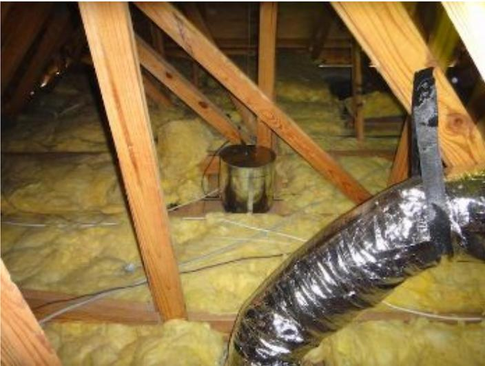
Showing new can light covers and new ductwork - before new insulation added.
