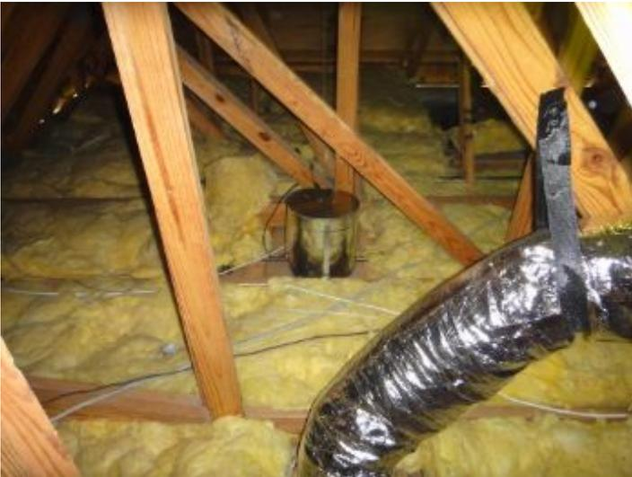
New light can covers - excellent - and new ducts, Area now full covered with insulation.
